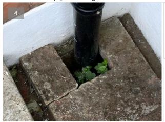
Gutters and downpipes are of uPVC material with no evidence of leaking joints or obvious signs of overflowing noted. They appeared intact but it was not raining at the time of inspection. Condition rating 1. No repair is currently needed. The property must be maintained in the normal way.
