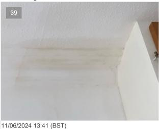
The ceilings have been covered with a heavy lining textured paper covering. Damp patches were viewed adjacent to the chimney breast at first floor level. Although it's not clear if the chimney stacks have been removed or if the dampness evident is historic. Removing this during redecoration may damage the plaster and you should plan for additional repairs. Condition rating 3. The defect is serious and/or needs to be repaired, replaced or investigated urgently.
