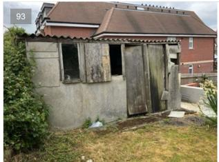
The outbuilding(s) comprising a timber/sheeting structures located at the rear. The roof is finished with corrugated roofing sheeting. The buildings appear poor condition and it would be more economical to demolish and rebuild opposed to considering repairs. Condition rating 2. A defect needs repairing or replacement but is not considered to be
