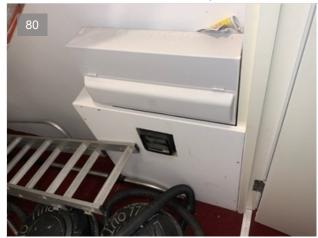
The property has a mains electricity supply. The electricity meter is located within an internal enclosure with the consumer unit. The supply is 60A/100A and a standard meter is installed. I saw no evidence that this electrical system has recently been inspected in the form of a test certificate. Condition rating 3. You should ask your legal adviser to request evidence of test certification.
