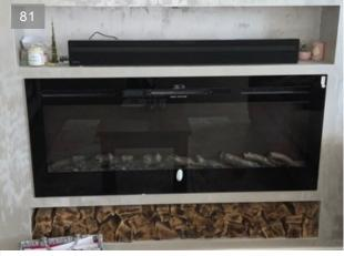
An electronic fire is located living room. The electric fireplace doesn't use air from the room for combustion, therefore, there is no need for open vents as required by the Building Regulations for gas fires. Condition rating 1. No repair is currently needed. The property must be maintained in the normal way.
