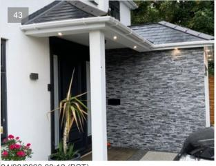
The porch is in a canopy arrangement and the roof is hipped and covered with tiles. The framing is made of timber in a suspended arrangement. There is a plastic gutter to disperse rainfall, although the downpipe is remote. It appears to be in a good condition with no evidence of rot or decay. Condition rating 1. No repair is currently needed. The property must be maintained in the normal way.
