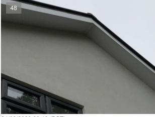
The external joinery/finishes made of uPVC appear reasonably flat and free from damage. These items are in good condition and should be relatively maintenance-free. Condition rating 1. No repair is currently needed. The property must be maintained in the normal way.
